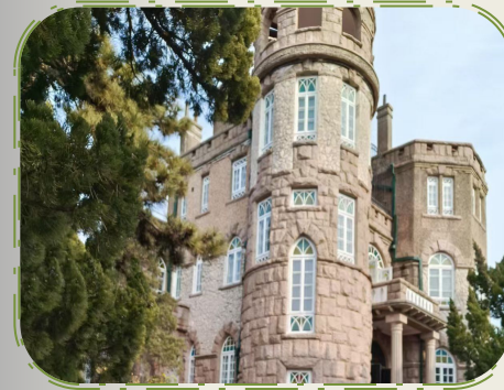
The Huashi House
